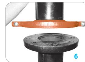
**Warning:** It is important to line up the bolt holes before bringing the two flanges together. Sliding the flanges into place will dislodge the gasket and cause leakage to occur. When using a flange insert, it is important that the insert is properly aligned with the gasket prior to tightening the bolts.
